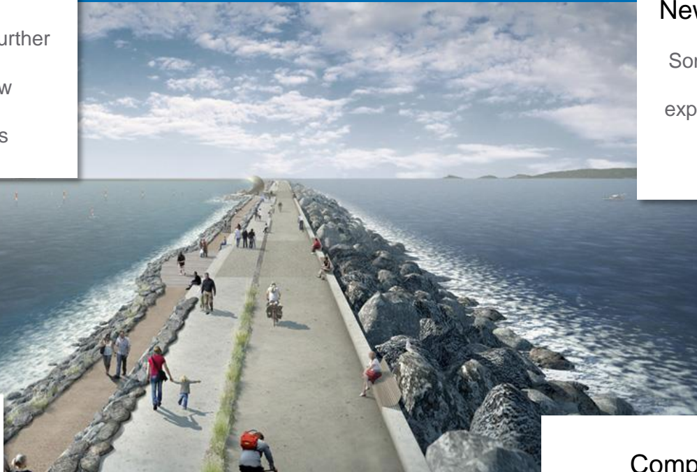
▲ The tidal lagoon hydropower plant in Swansea Bay, Wales, will have a total capacity of 320 megawatts.
